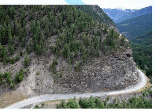
Photo of a bluff requiring rock slope remediation. Part of a government remediation project, this photo will be one of many used to calculate the mesh area and other requirements.
