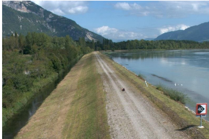
Figure 1 : Aerial view of a dike
