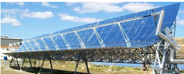
Figure 2: EuroTrough line focussing collector module
