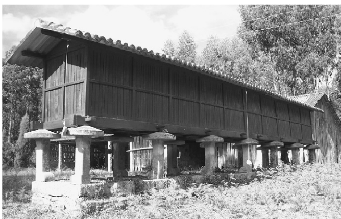
Fig. 2. Photograph of the hórreo . Two stones suspended by ropes and acting as plumb lines can be noticed.
