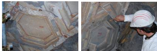
Figure 13. Detail of a in-situ consolidation and restoration
