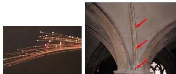
Figure 17. POF sensor placed to check the deformations
