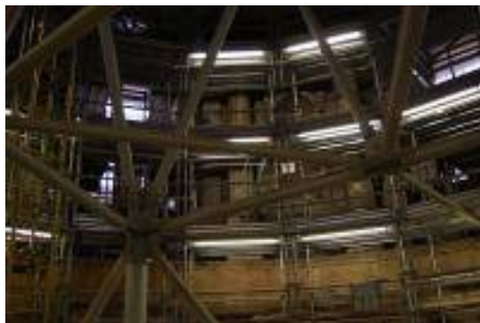
Figure 4. Metallic scaffolds used to ensure the structural stability
