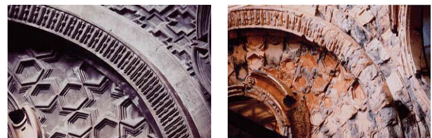
Figure 5. Decorative elements before and after the fire
