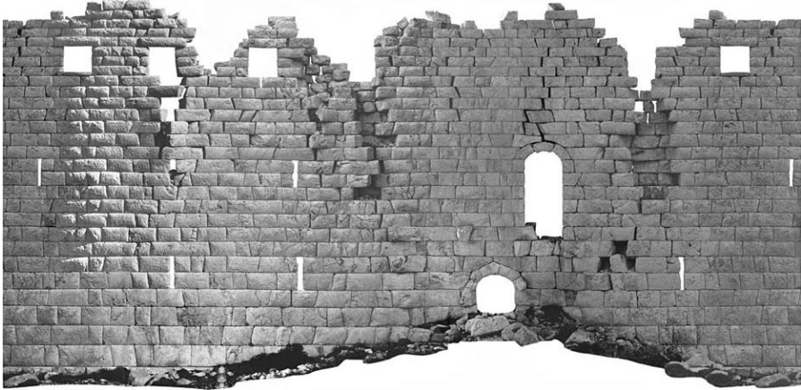
FIG. 4. Final raster development of the cylindrical Drakanos tower (a total of 17 “unwrapped” images have been mosaicked).
