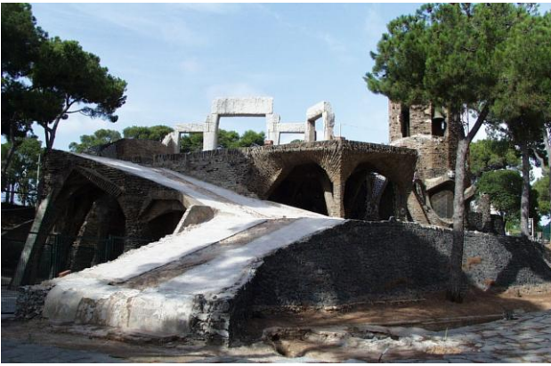
Fig. 3. Entrance facade of the crypt
