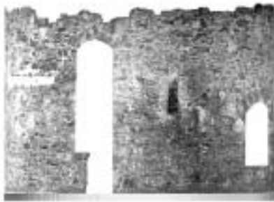
Fig. 5: a side view automatically derived from a cylindrical orthophoto.
