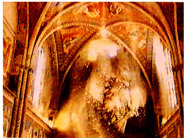
Figure 13. Collapse of the ceiling of the Assisi Basilica during the earthquake of 27 September 1997 [6]
