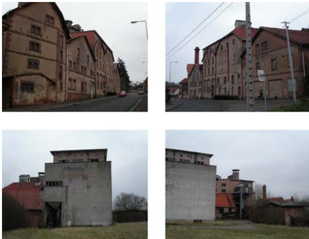
Figure 3. Ingwiller old malt house
