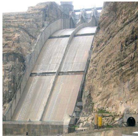
Figure 1: Spillover of Marun dam
