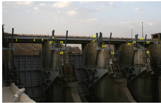
Figure 6: Control points position on the spillover
