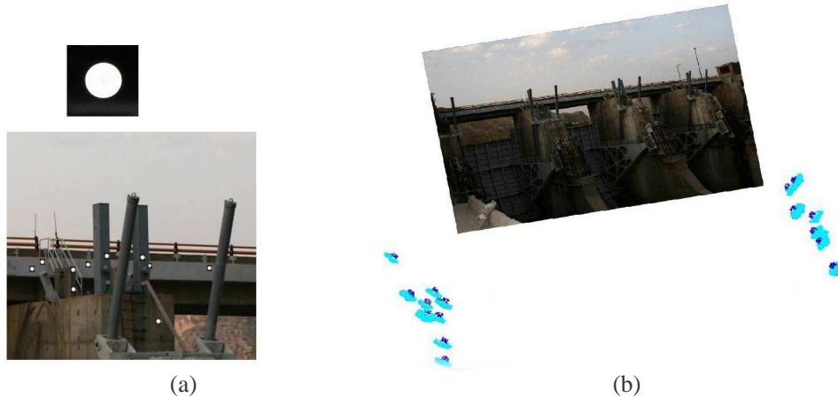
Figure 2: (a) Targets on spillover, (b) Photogrammetric network design view
