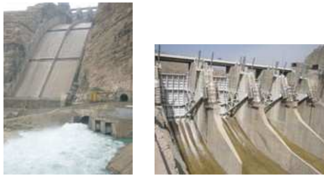
Figure 1: spillover of Marun dam
