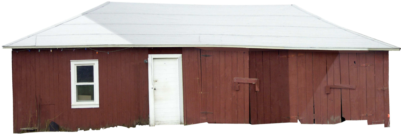
Orthophoto of facade
